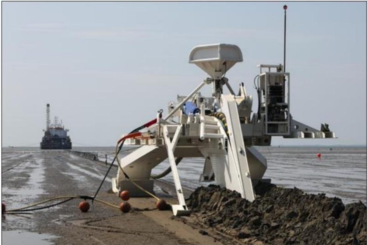
Plate 3-1: Example of a Non-Displacement Cable Plough (Photo Credit: Boskalis)
